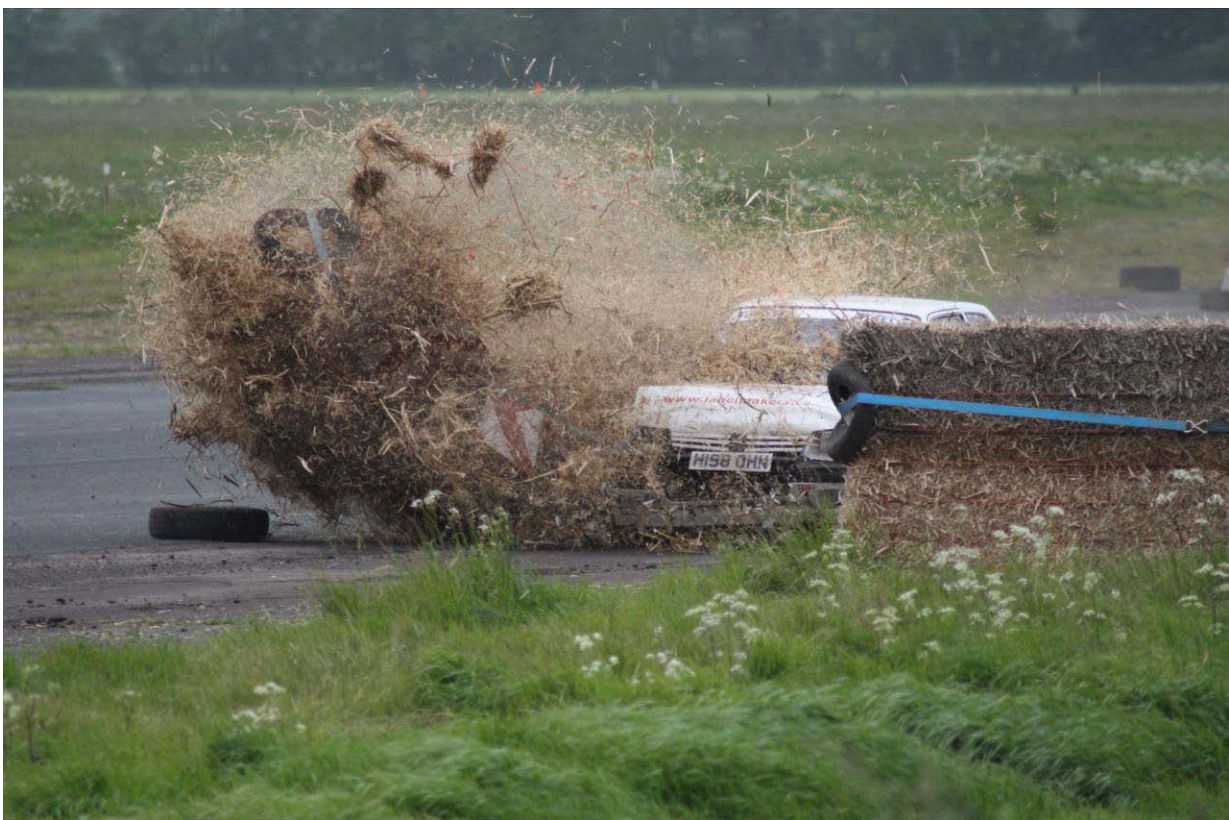
Chicane demolition on the John Overend Photo courtesy of Kim Barnes
